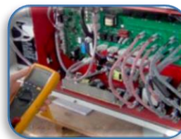
Checking the Electrical Panel
